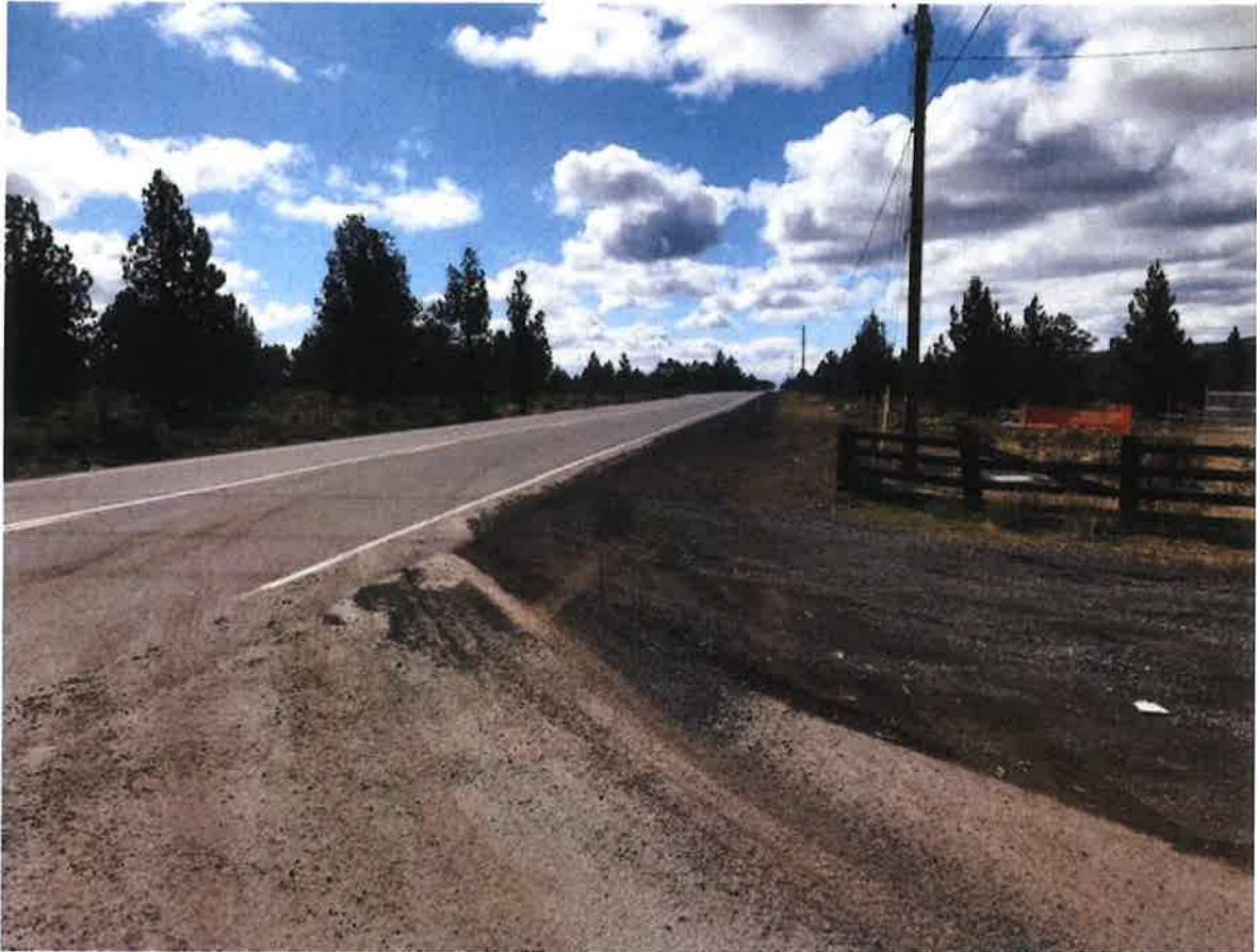
Figure 6. Por-Tay access facing south along Millican Road.
