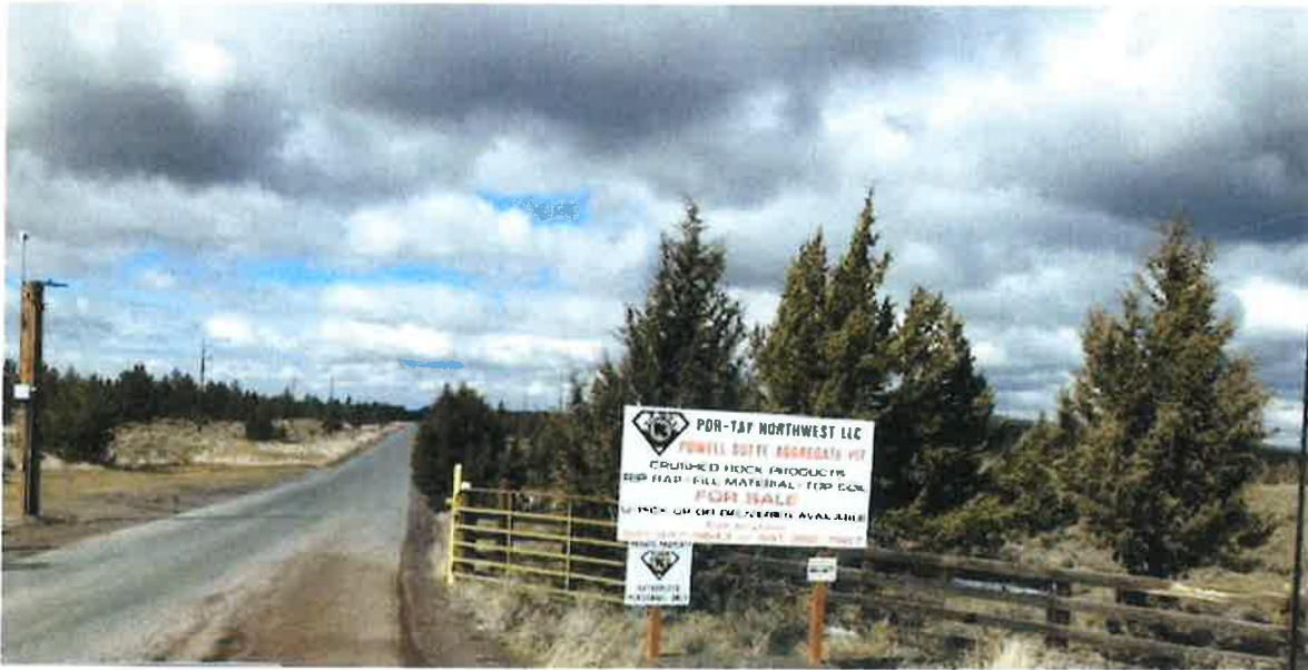
Figure 3. Existing Por-Tay Quarry Access from Millican Road.
