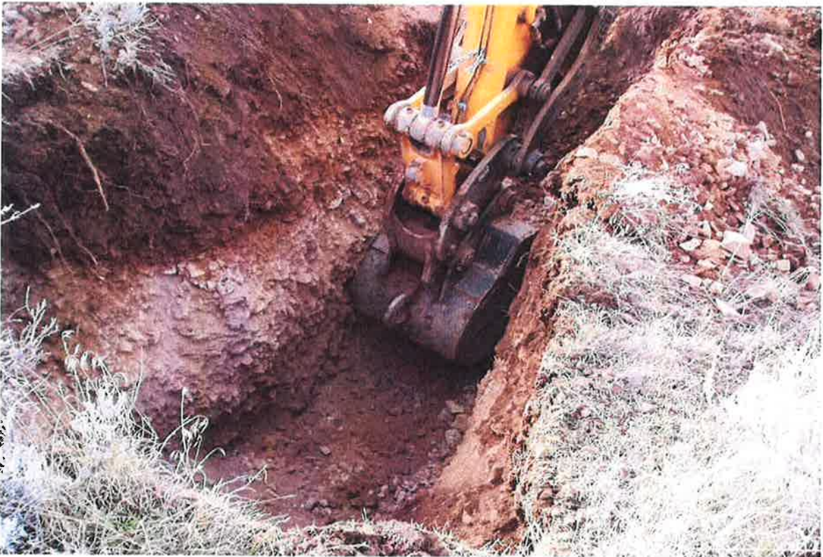
Test Pit TP-03
