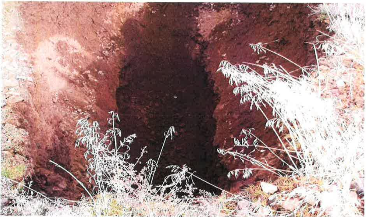
Test Pit TP-05
