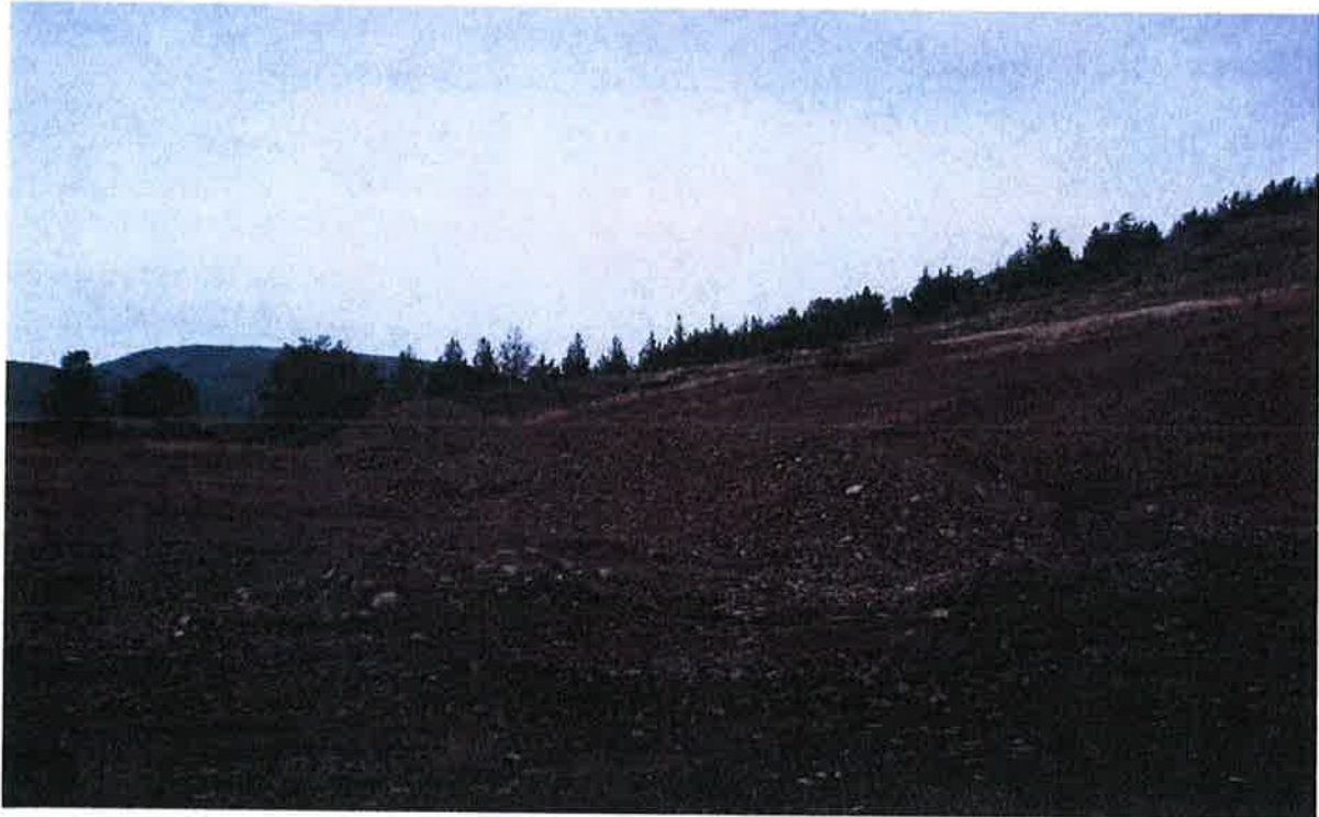
Small piles of excavated material, north portion of lower terrace
