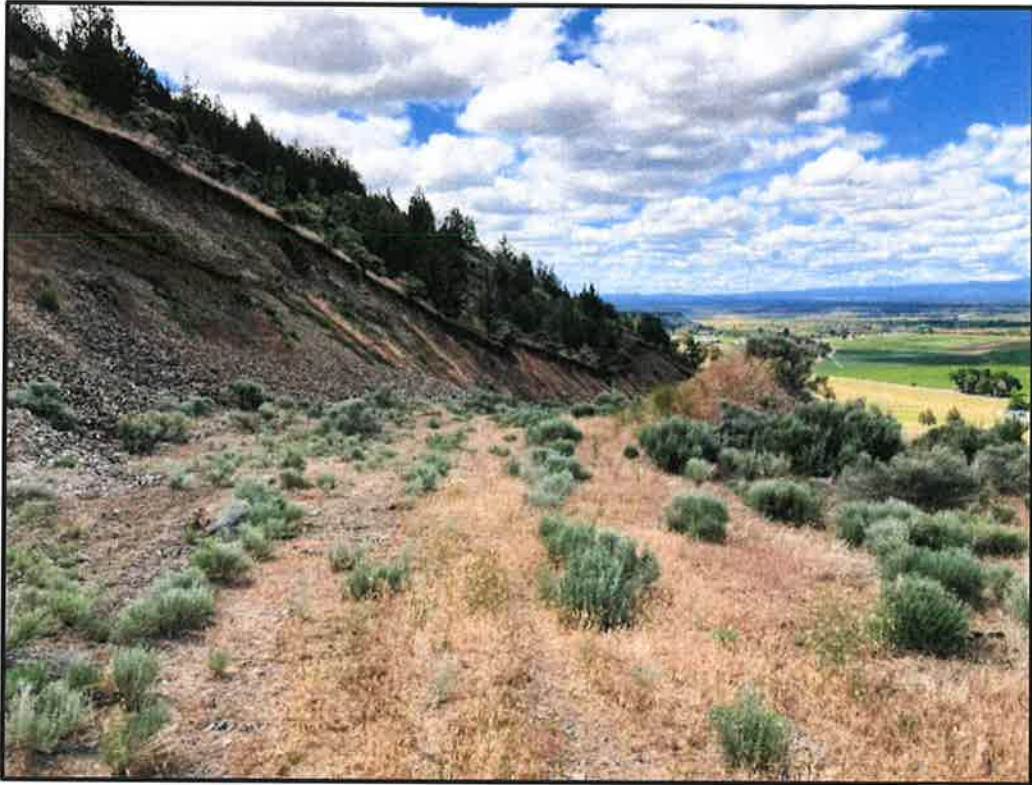
View looking southwest at existing road cut.
