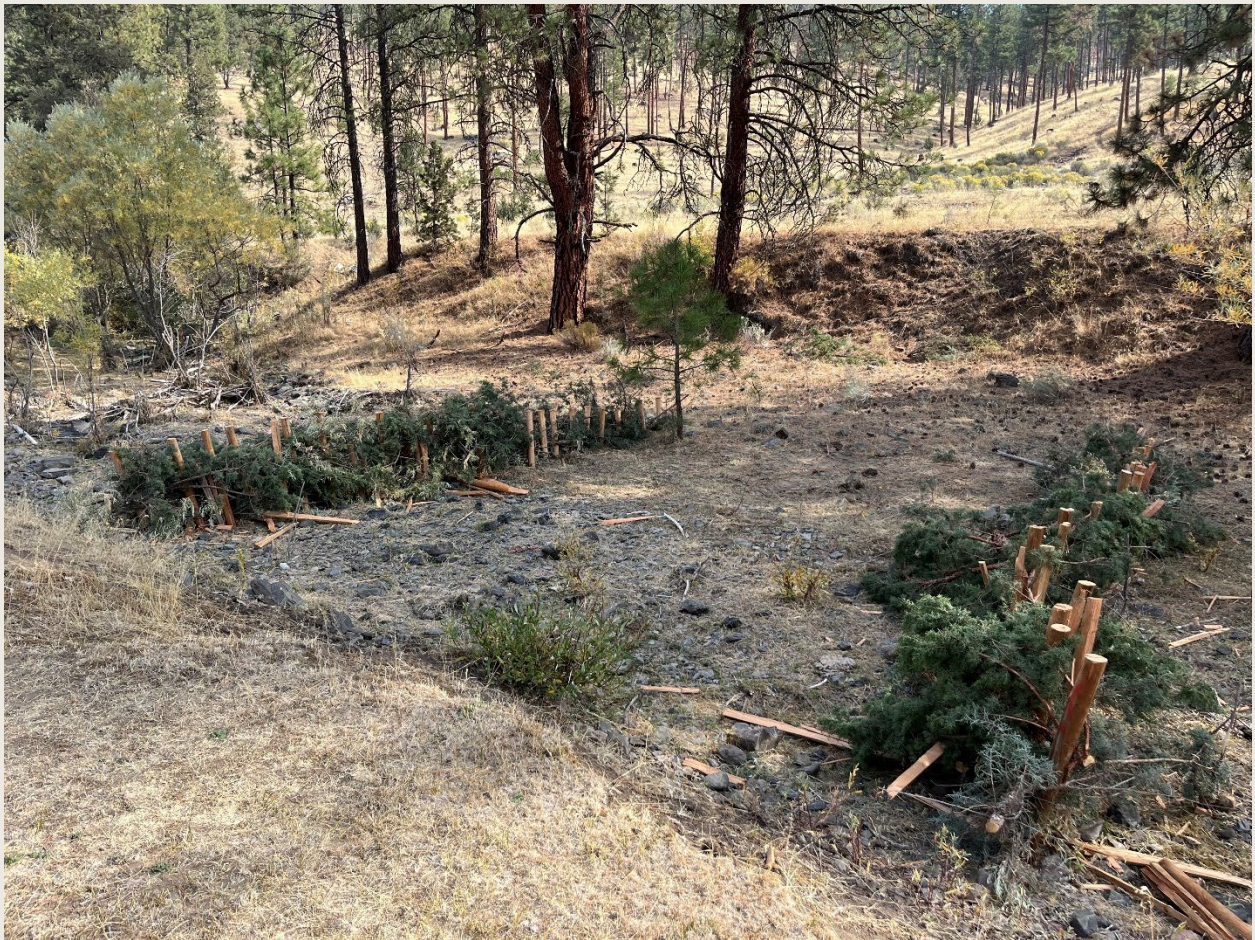
Instream Beaver Dam Analog Project on the Foley Butte project 2024
