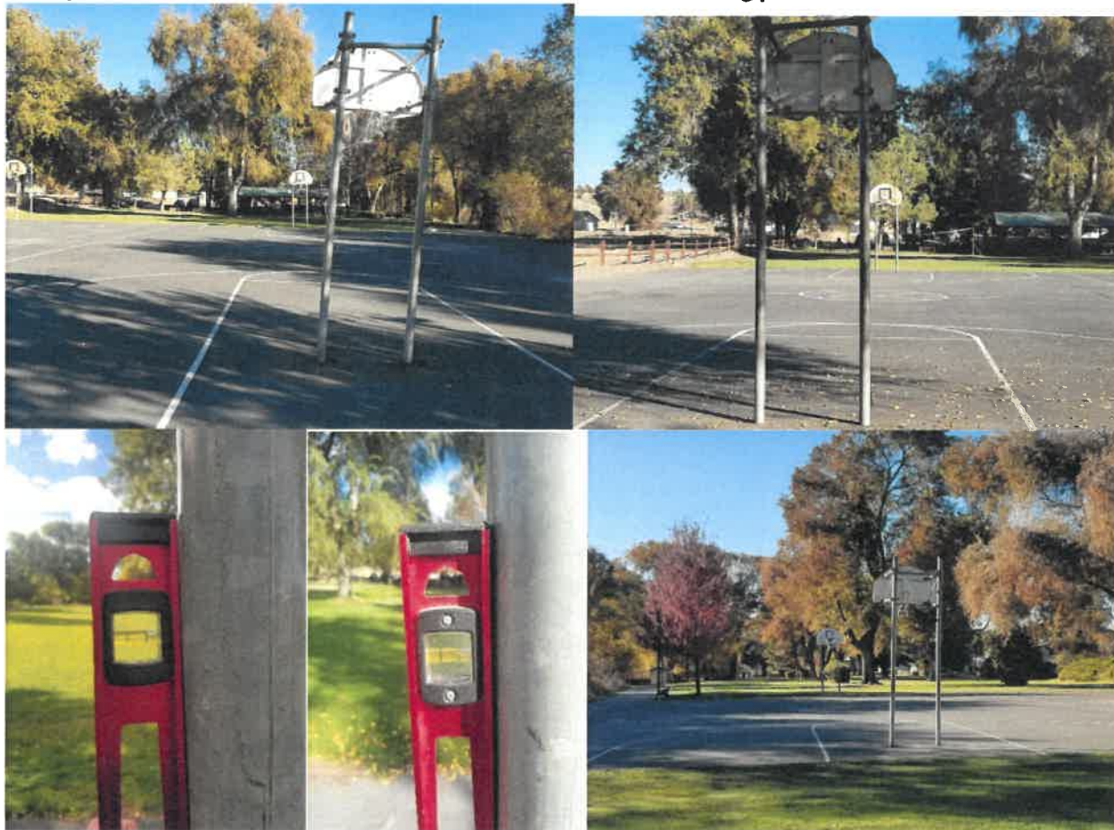
Examples of standards conditions – Lack of vertical trueness or being plumb
